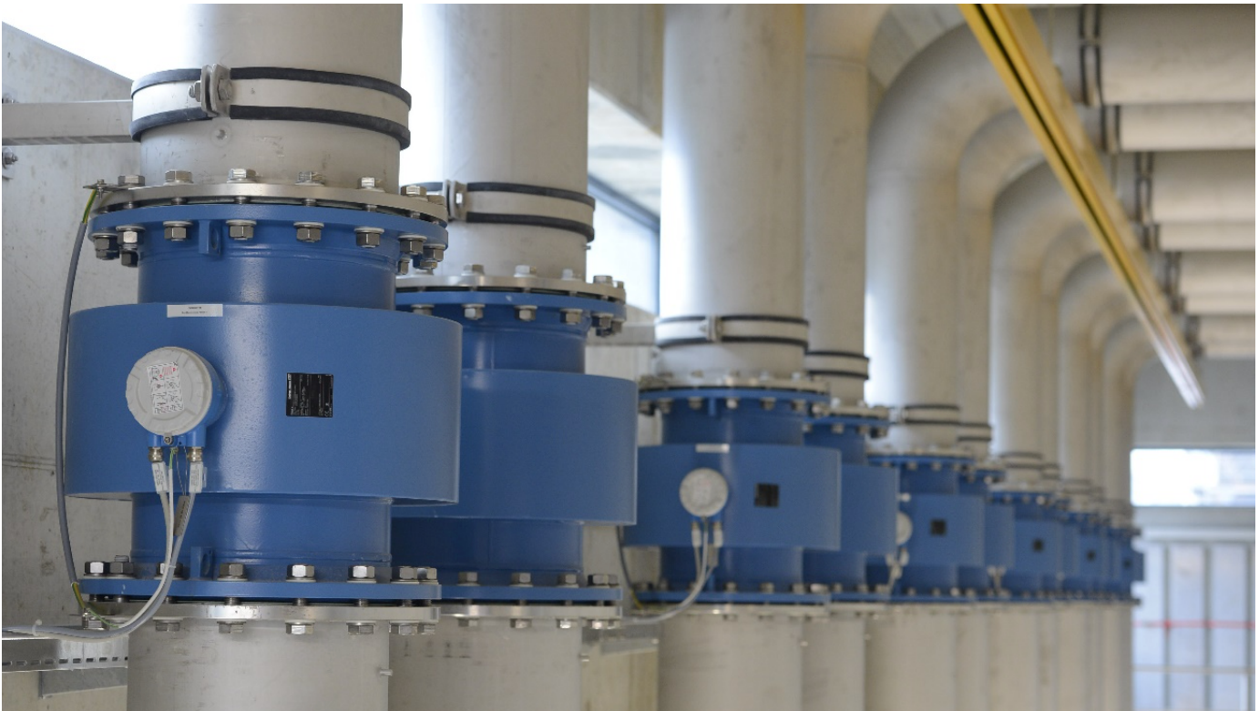
Figure 1: Endress+Hauser’s Proline Promag W electromagnetic flowmeters transmit multiple variables and instrument diagnostic data via HART, WirelessHART, and Bluetooth.
