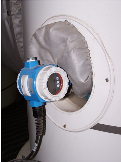
Cerabar S PMC71 absolute pressure transmitter mounted on distillation column
