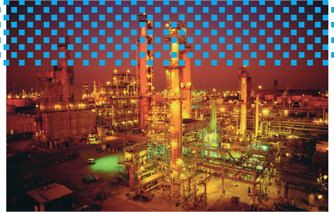
Typical chemical plant
