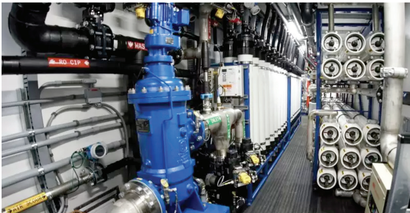
MPW Industrial Services' mobile ultrafiltration/reverse osmosis water filtration system
