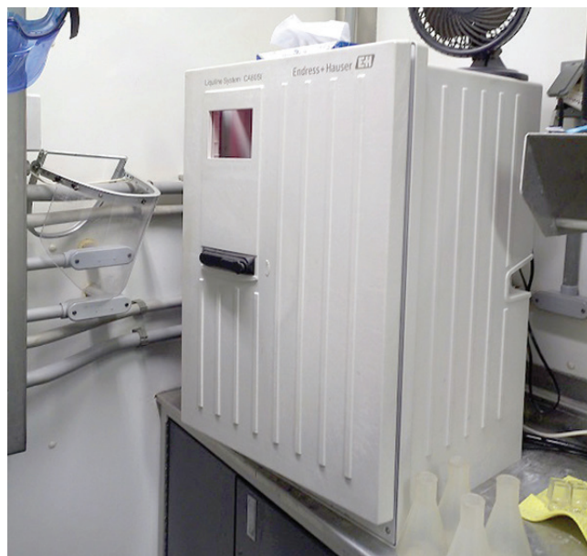
Endress+Hauser's Liquiline System CA80SI silica analyzer on-site at MPW's Hebron, Ohio facility
