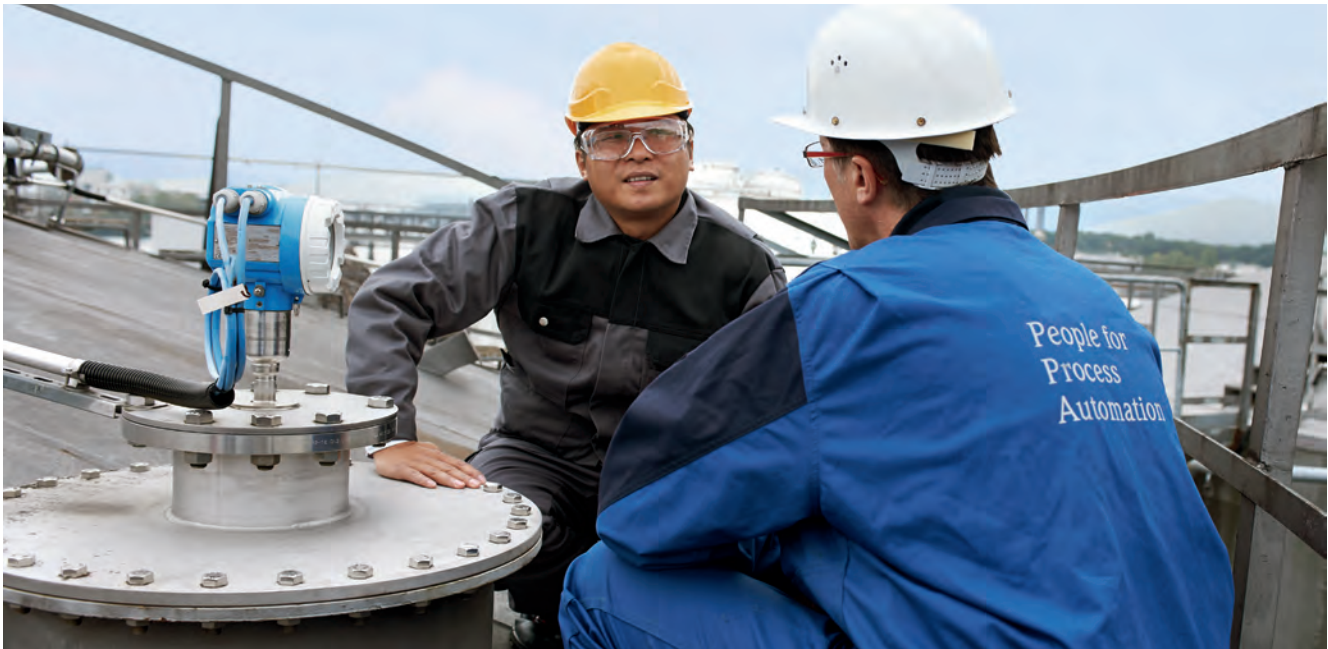
FIGURE 1. Radar level instruments have the necessary accuracy for custody transfer applications.
