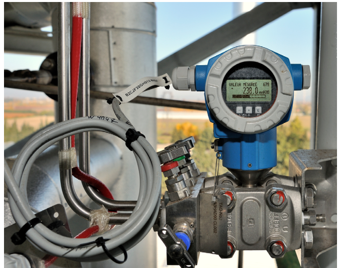
Figure 2: Five-valve manifold (to left of transmitter) is used to isolate a pressure instrument's sensor so it can be removed from the line, re-zeroed or calibrated.
